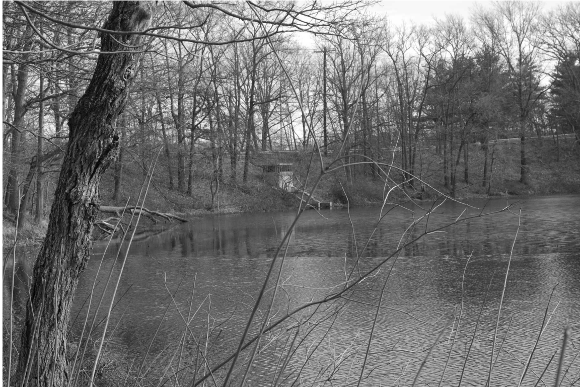
Butterfield dam, showing inlet structure in center, and large trees growing in the dam.
