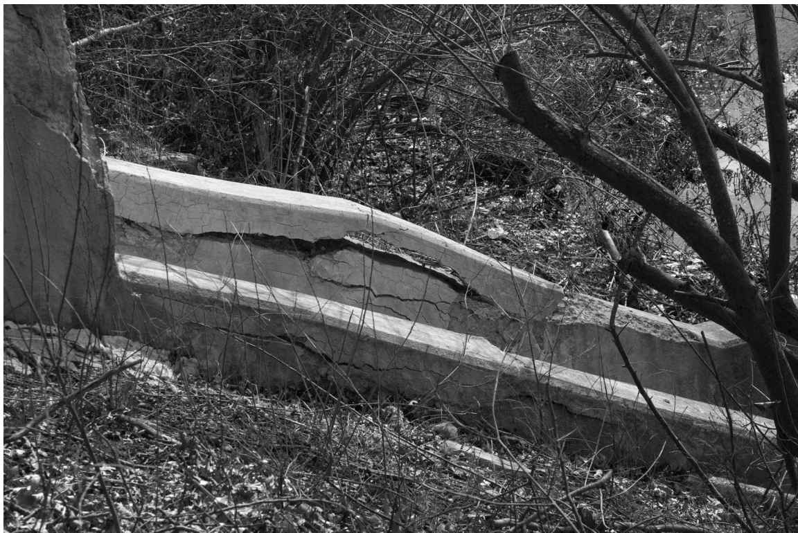
Close-up of some of the inlet structure's damaged concrete to be repaired under Phase I funding. There is extensive cracking of all parts of the structure and exposed rebar.
